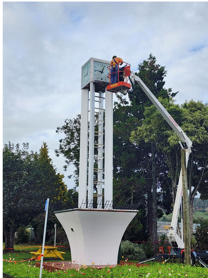
Te Kuiti town clock repair April 2023
