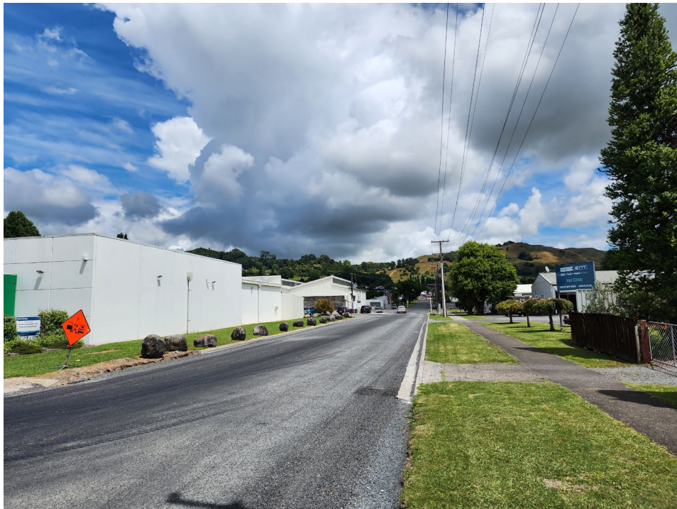
Rehabilitation of Seddon Street, Te Kuiti
